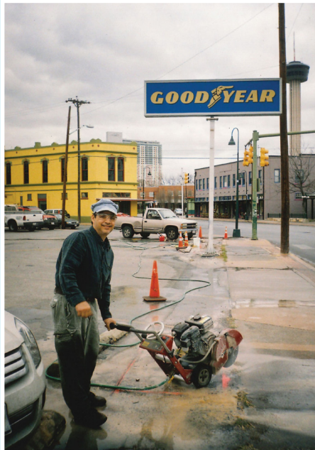
02/07/09 | Oscar Alvarado cutting holes in parking lot at Goodyear store at S. St. Mary's and Alamo for five trees
